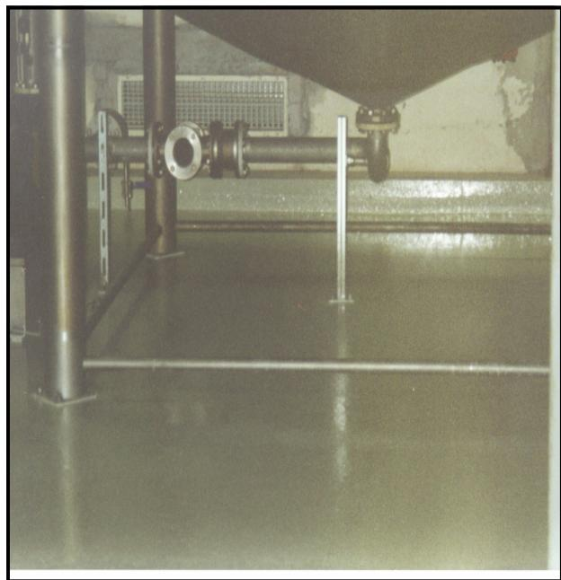
The floor surface was prepared by blast cleaning.
